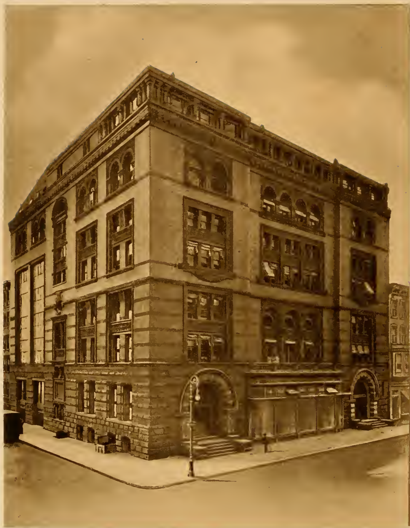
TIFFANY STUDIOS SHOWROOMS AND GENERAL OFFICES
