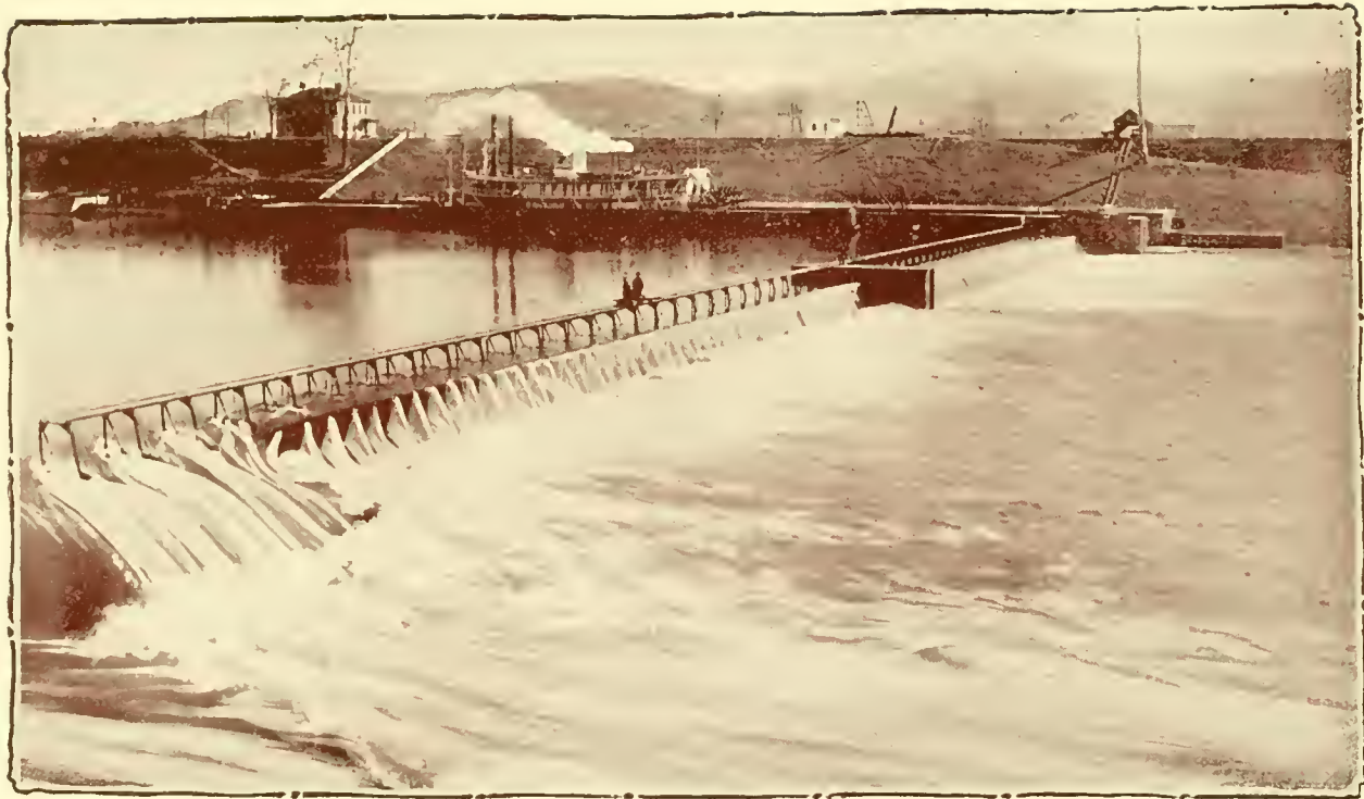
Lock and Dam No. 6. Showing the Dam up . View taken from the abutment side. Tow-boat with empty coal barges just passing out of the lock. Part of the Weir of the dam is open, a few of the weir wickets and bridge trestles next to the abutment (the abutment is not shown in the picture), having been put down on account of a small rise in the river.
